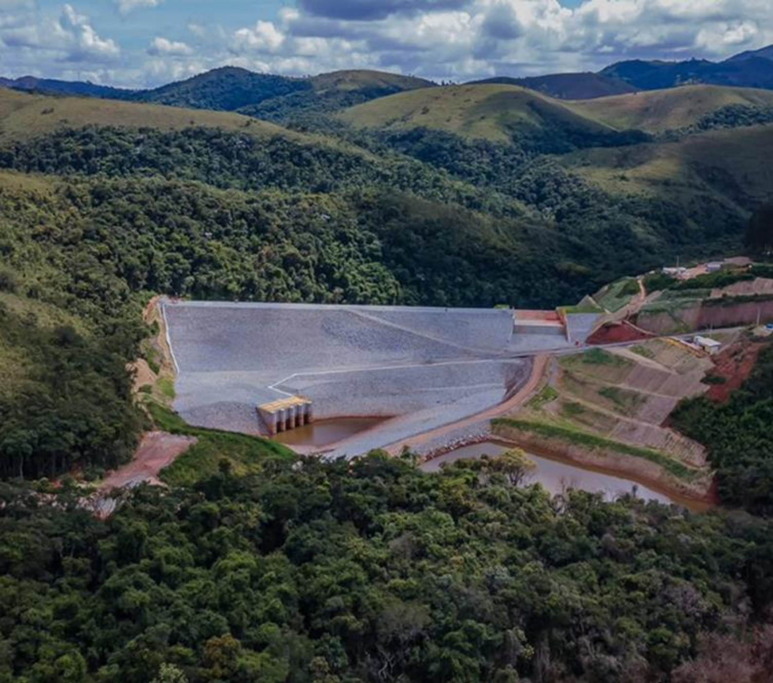
B3/B4 back-up dam, delivered in 4Q20
