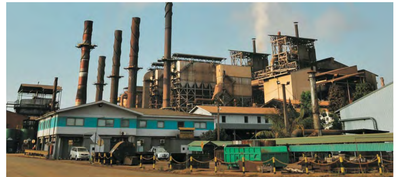
Area Vale | Vale Area
